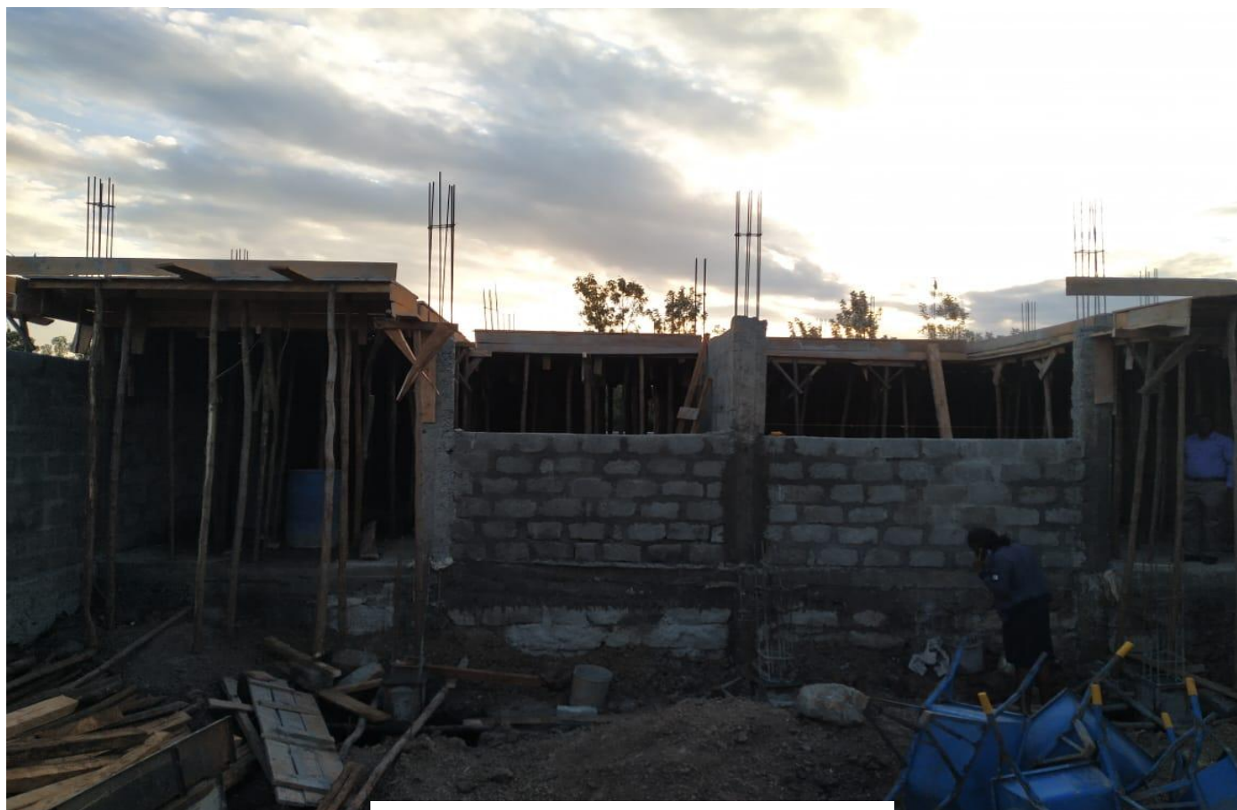
CONSTRUCTION OF A FIVE STORY BUILDING IN RUIRU
